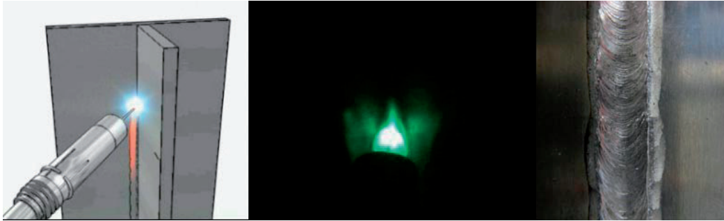
Figure. Aluminium position welding.
